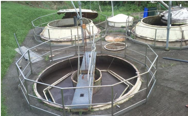
Figure 2.1 - Vue de la station
